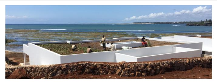
In conventional roof gardens, bulky & heavy graded stone filter layers have been replaced with a HDPE cuspated sheet with a nonwoven geotextile bonded to one side. The nonwoven geotextile provides soil separation and filtration while the HDPE core provides a structural drainage system and added protection to the waterproofing membrane.
